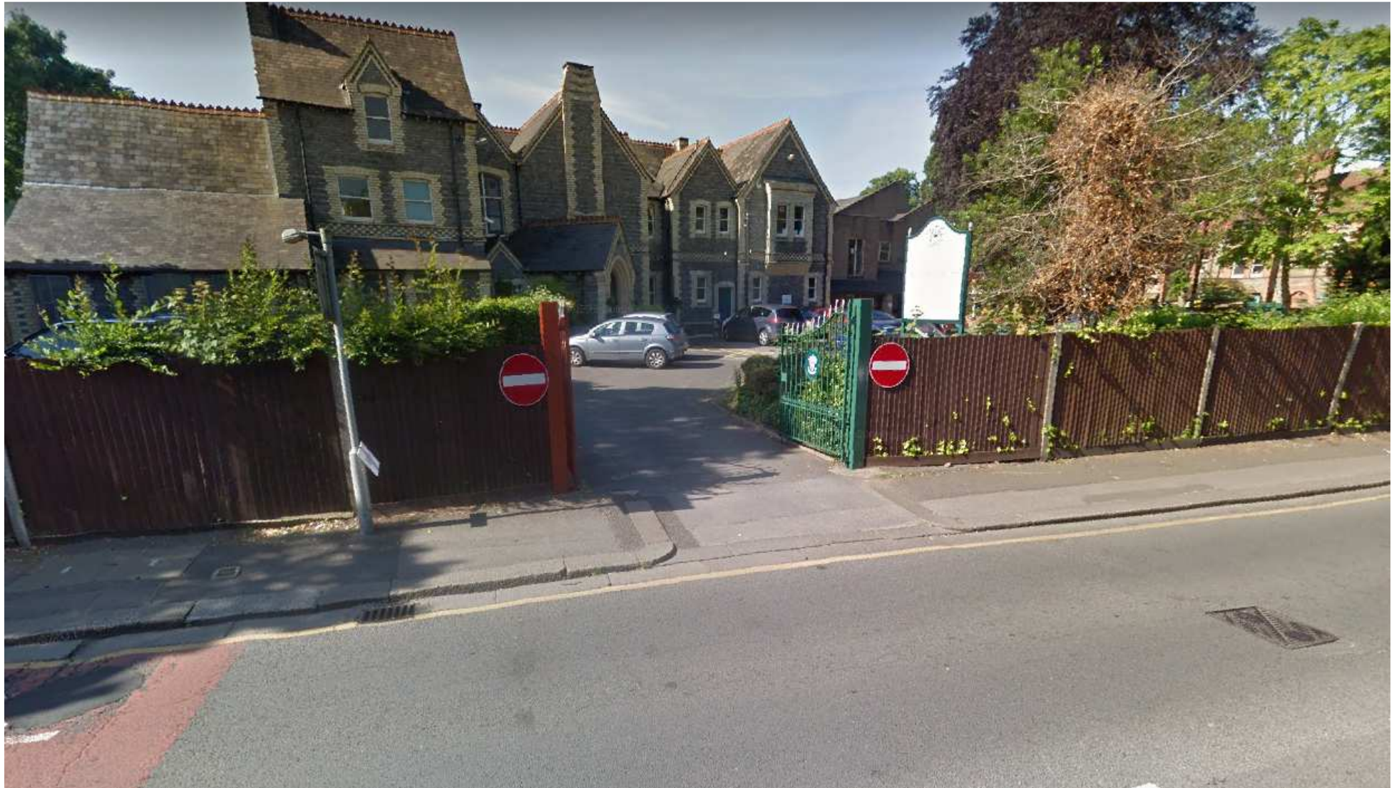
Image 1 - Existing dropped kerb access located onto Christchurch Road
