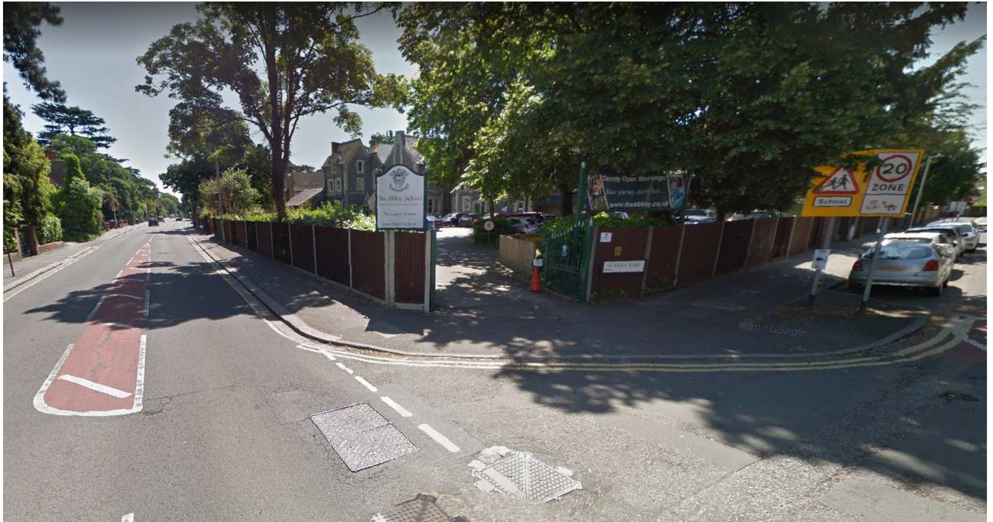
Image 2 - Existing dropped kerb access located on the radii of the Christchurch Road / Vicarage Road junction
