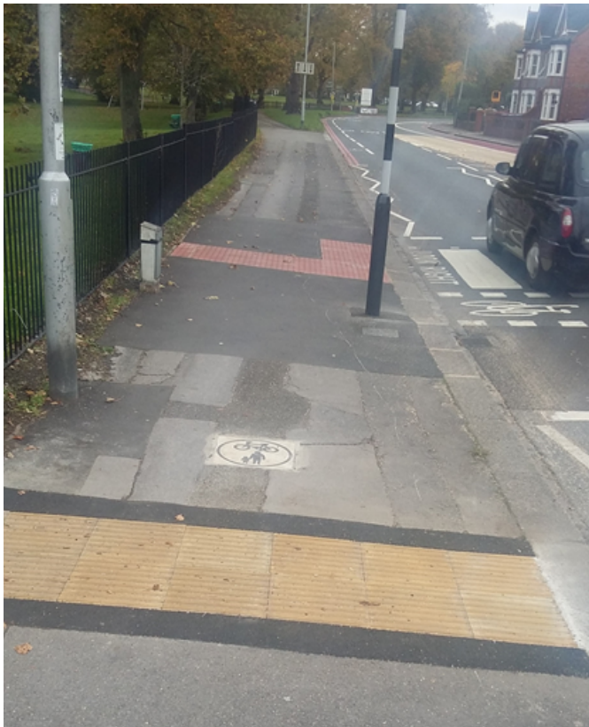
Figure 4 – Corduroy paving on approach to parallel crossing
